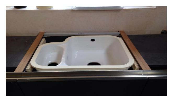
For other undermounted sinks they should be installed in a solid top like below and routered so 1mm lower than the level of the sides of the carcase
